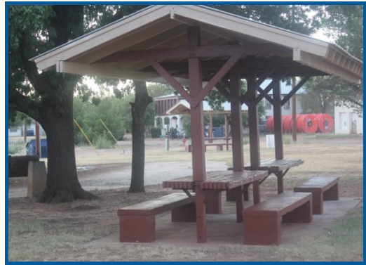
The City of Spur used their grant to make improvements to Rickels Park in Spur.
